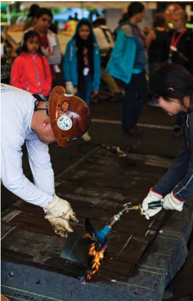
A middle school girl learns the "torch down" roofing technique in a workshop with the Oregon & SW Washington Roofers & Waterproofers. Photo by Lindsay Cimina Photography.
